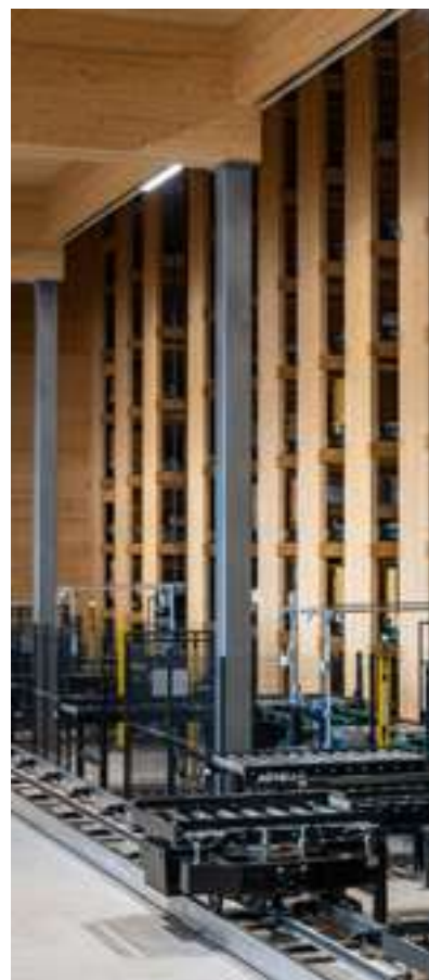
The first automated free-standing warehouse in Italy with a wooden structure. Cortaccia (Bolzano)
